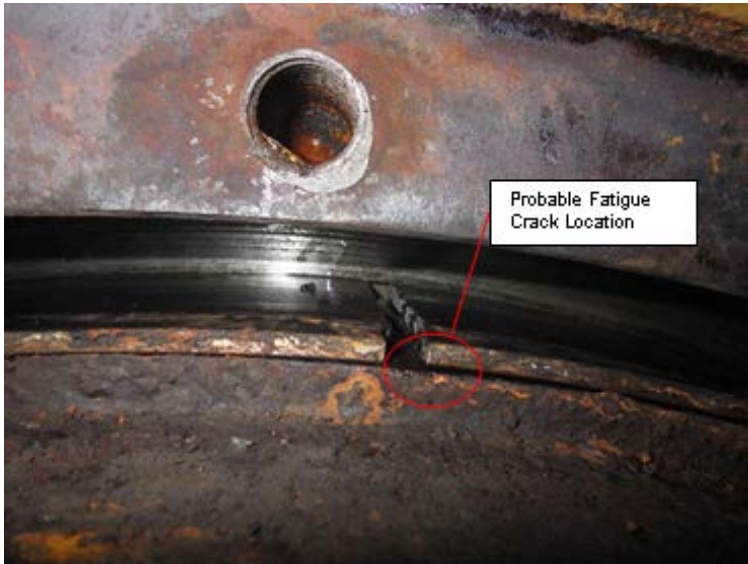
Photo 1. Broken sleeve as found in the blade packing box
